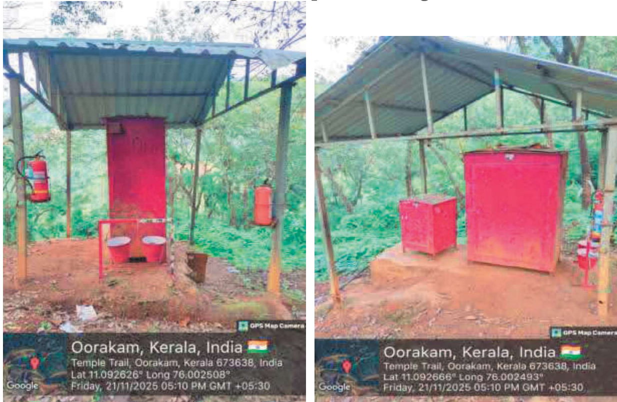
Figure 9 :Explosive storage area
